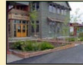
Vegetated Infiltration Basin
